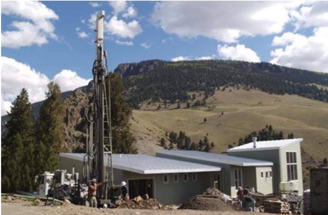
Drilling costs have averaged \$23.00/foot in Creede America. All 6 operational systems provide 100% of domestic heat. 4 systems also provide 100% of domestic hot water. The largest systems in Creede have four 300' boreholes for a total drilling cost of \$27,600.00. The smallest system has two 300' boreholes and cost \$13,800.00 to install.
